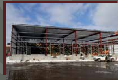
New Center Stamping Building Expansion
