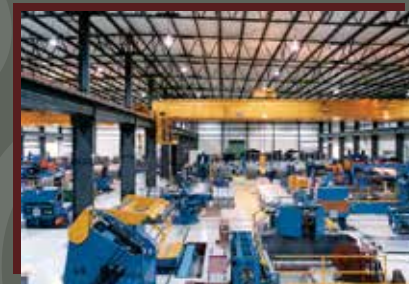
Kenwal Steel 200,000 SF Steel Facility
