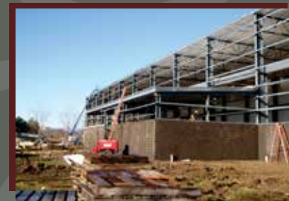
Grand Rapids Building Expansion
