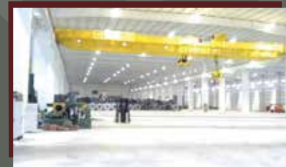
Romulus 230,000 SF Steel Facility
